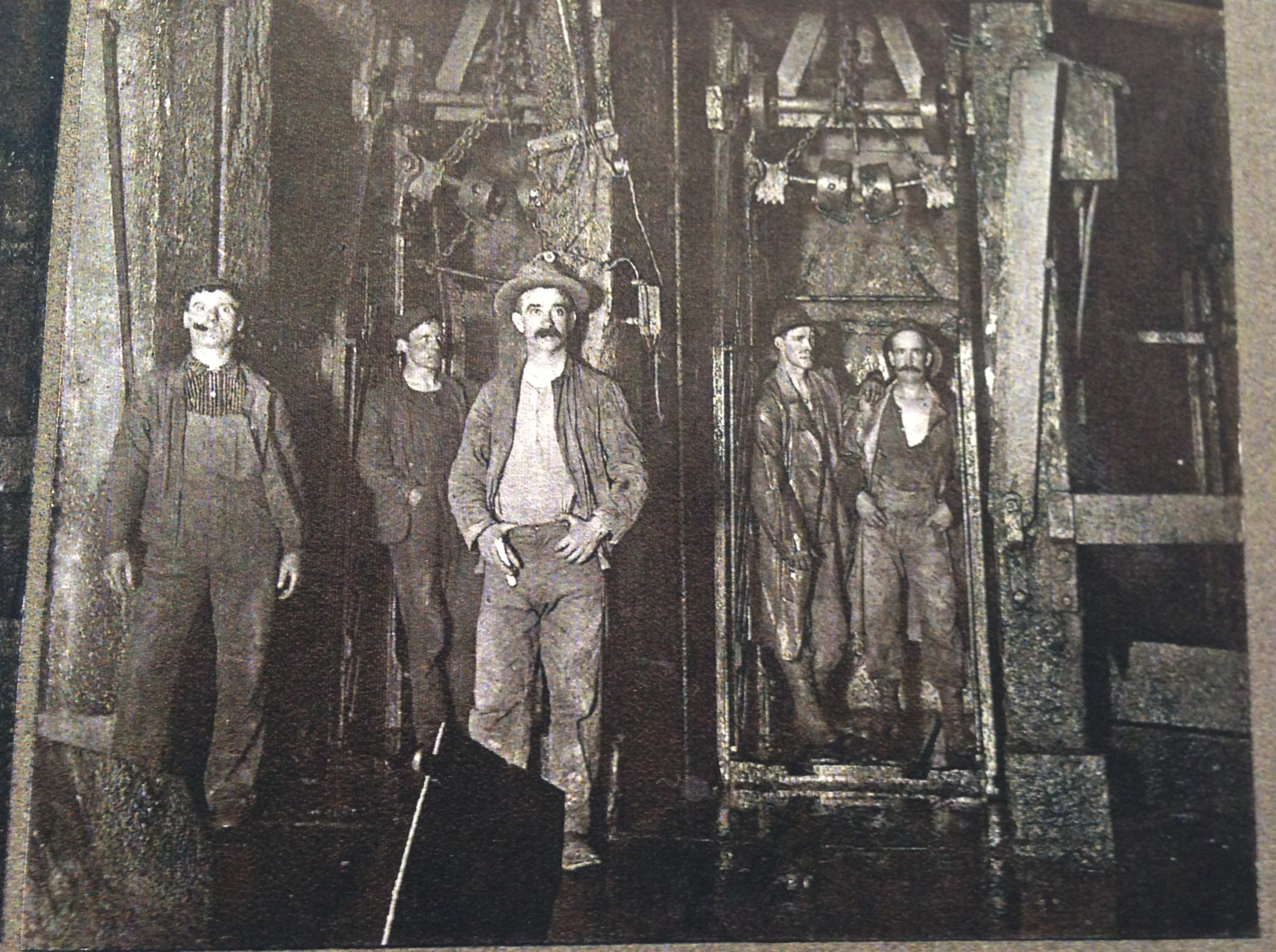
327. Station at 1600 level in Original Mine, Butte
